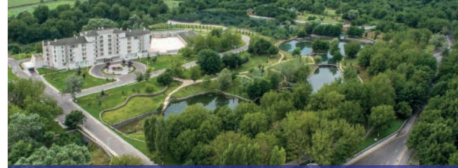
Turizm / Tourism Azerbaycan / Azerbaijan Qafgaz Yengice Termal Otel Qafgaz Yengice Thermal Hotel Adet /Piece - Güç /Power : 2 x 1125kVA
